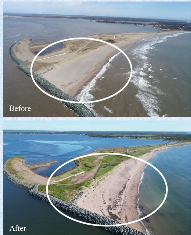
A coastal area before and after a sand engine was built in Shippagan, New Brunswick. Photo credit: Courtesy of CBWES
