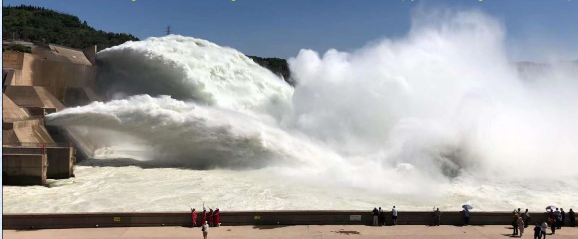
Flow and Sediment Regulation in Xiaolangdi Reservoir, the Yellow River (by Enhui Jiang, June 28, 2022)
