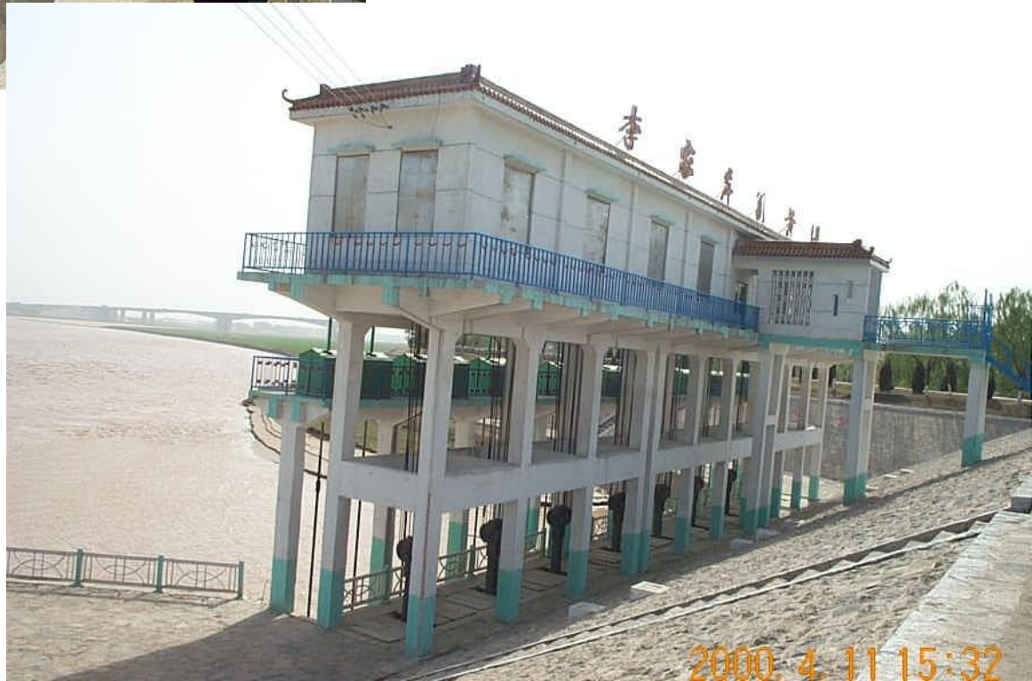
Lijia-an flood diversion gate: 150\text{m}^3/\text{s}
