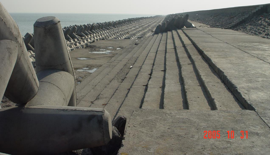
Breakwater and levees to protect the new created land at the new river delta
