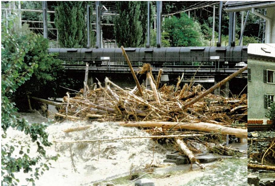
Blocked water intake of the water power station Massaboden
