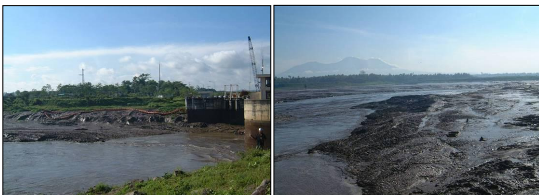
Figure 3 Sedimentation in Wlingi Reservoir
