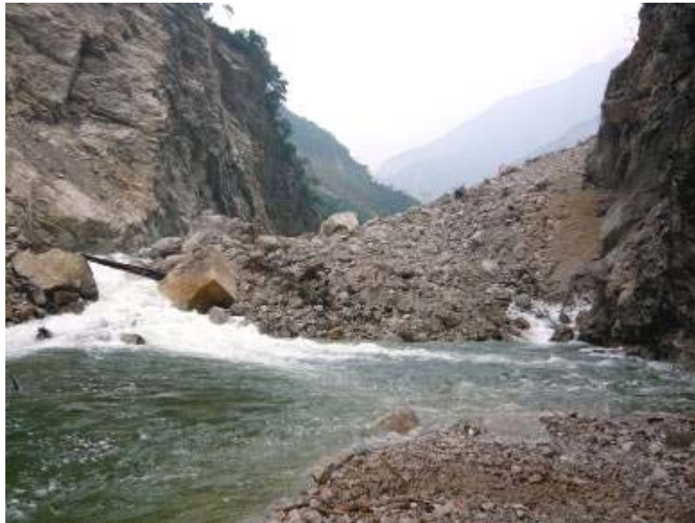
Figure 8 Clear seepage and overspill flows through a landslide dam on the Mianyuan River.
