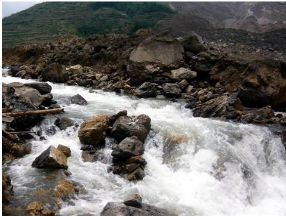
Figure 6 Preliminarily developed step-pool system in the spillway of a landslide dam on the Qingzhu River
