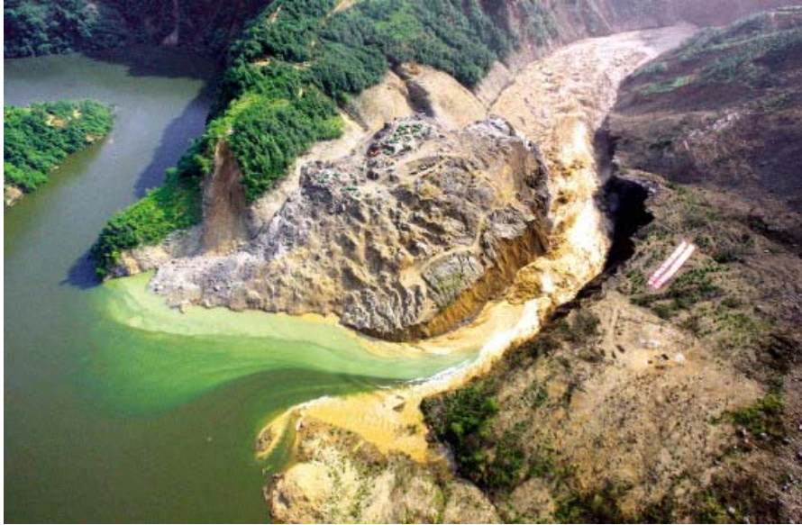
Figure 9 Lake water flows through the enlarged spillway from the Tangjiashan quake lake and scours the landslide dam.
