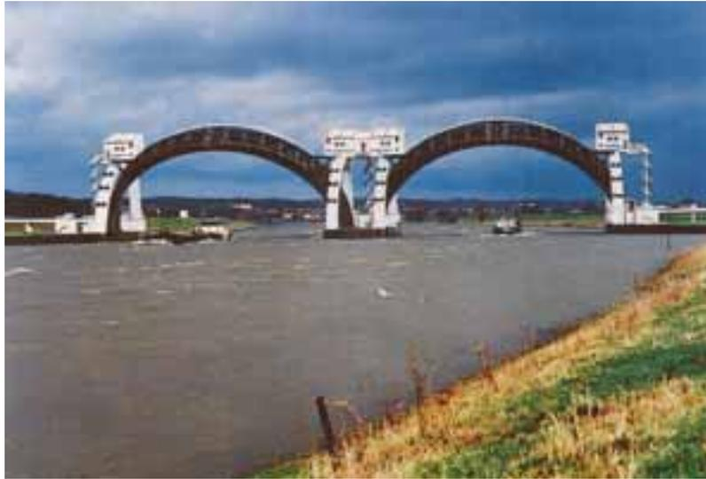
Fig. 9 The weir at Driel in the Lower Rhine. The weir directs water to the north or let it pass to the west of the country.
