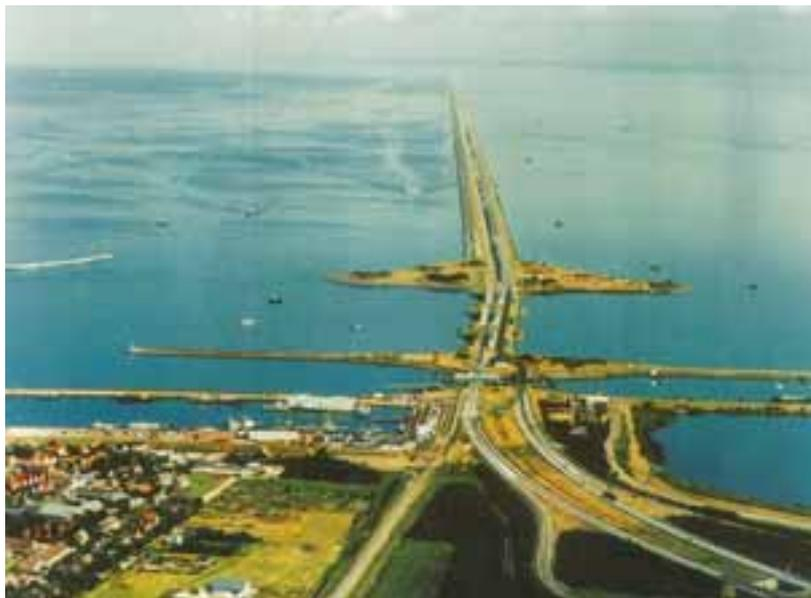
Fig. 10 The 32 km long main dam separates the Wadden Sea from the fresh water of Lake IJssel.
