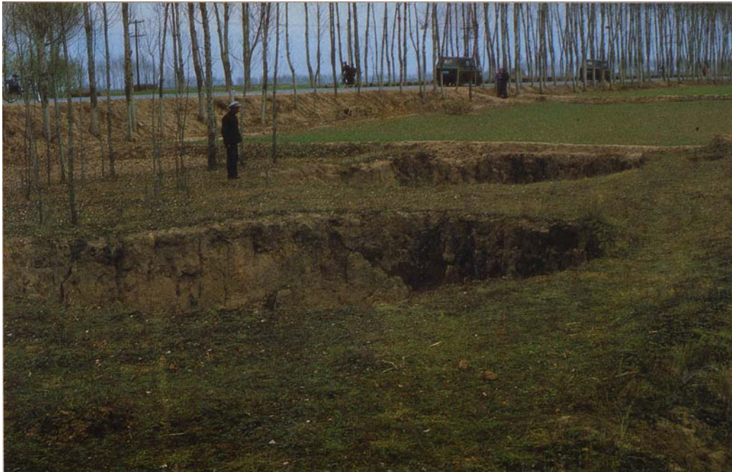
Photo5 Concealed Erosion - Funnel Erosion
