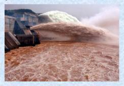
Water and sediment regulations is using reservoir storage capacity and man-made flood to scour riverbed, thereby reducing river siltation and even balancing the erosion and deposition so as to curb the riverbed. (Edited and translated by Liang Jun, People's Daily Online)
