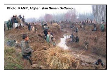
Figure 2B – Farmers de-silting the Char Dara irrigation canal in northeastern Afghanistan.
