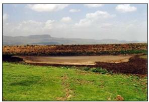
Figure 11C – Example of sedimentation in Ethiopian Reservoir (Migae reservoir)
