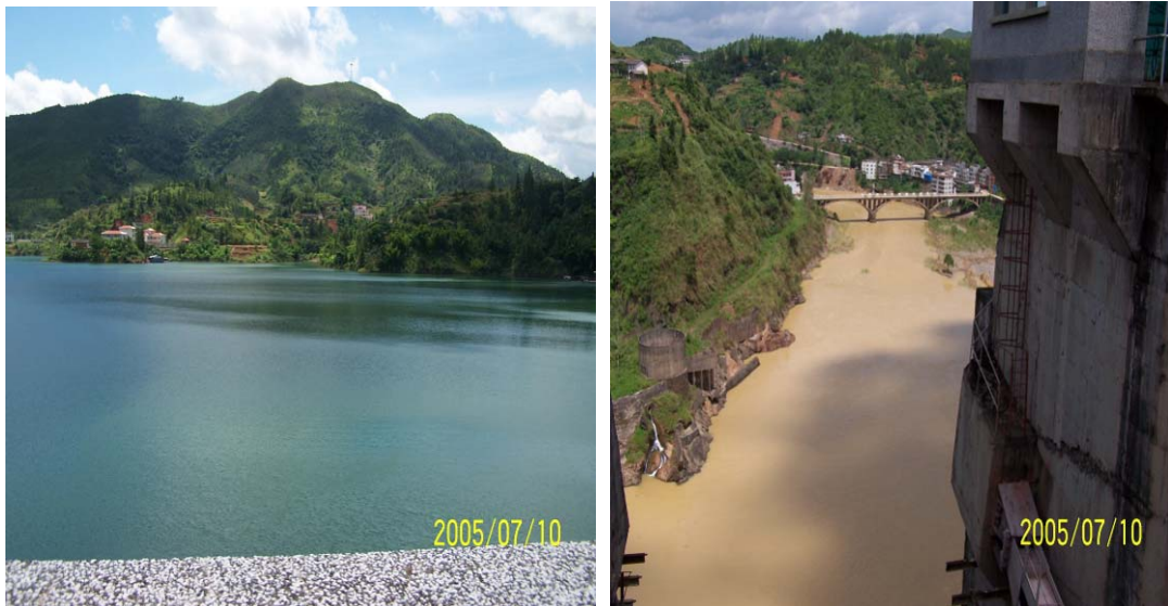
Fig. 2.4 Up (left) and downstream (right) views of the Fengshuba Dam
