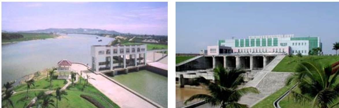
Picture 7 Water diversion works and pumping station of the Dongguan-Shenzhen Water Supply Project
